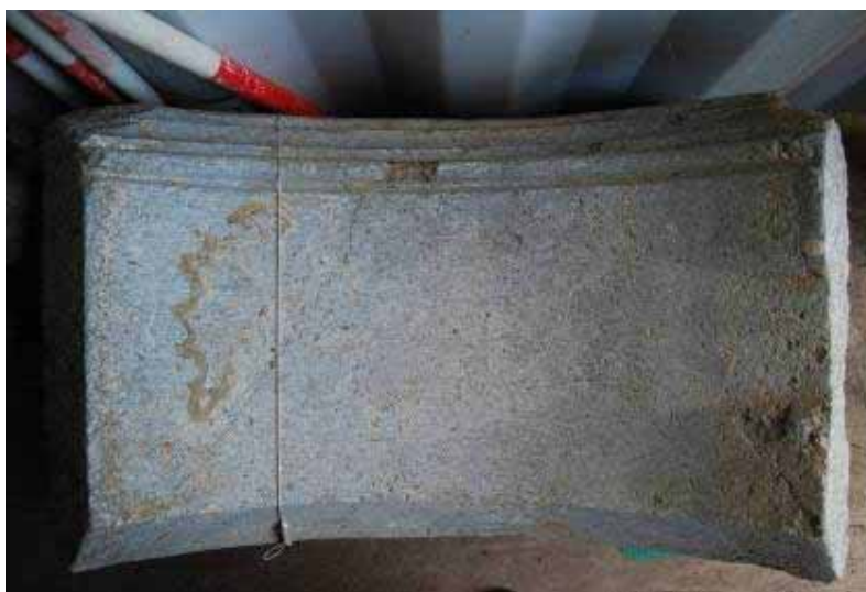
Plate 22: Underside of arch stone from cloister arcade, this would have been one stone from the arch which would have been composed of two of these, and possibly a third keystone
